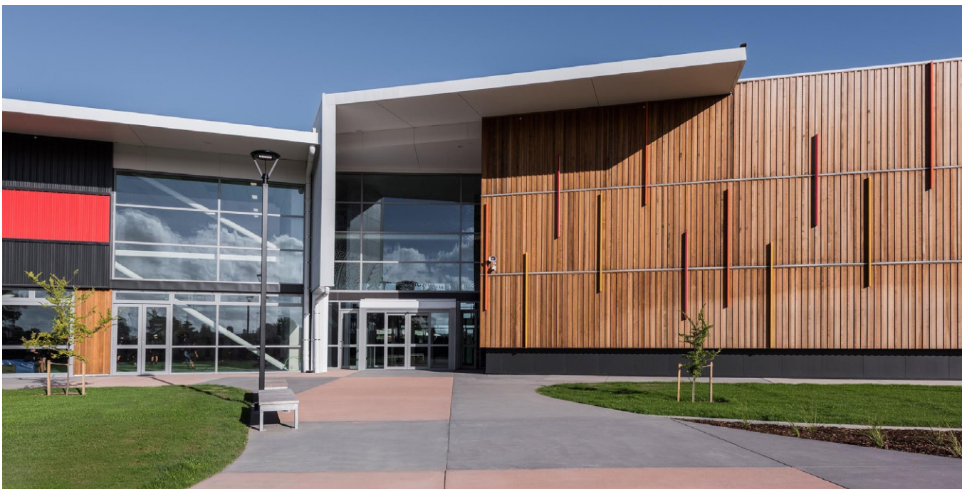
Figure 24: Haeata Community Campus entrance.
