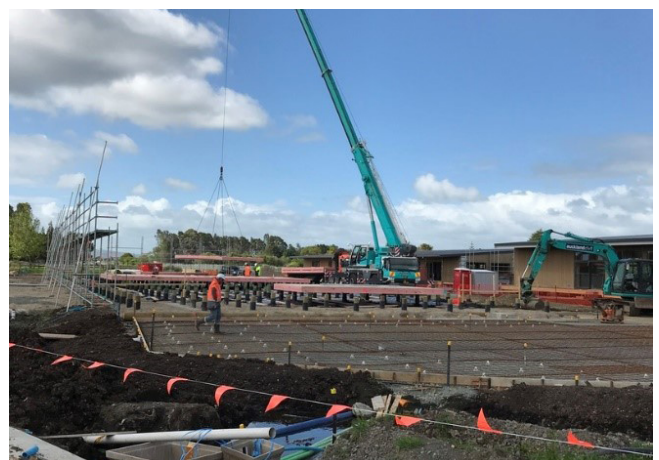
Kauri Flats School Construction Zone.
