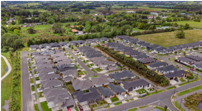
Birds eye view of homes in Kauri Flats showing high density housing with small outdoor spaces. (Image source: Cappella https://cappella.co.nz/work/kauri-flats-takanini )
